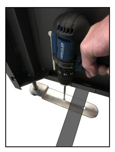
Remove 8 screws holding lift bars, and dispose of lift bars
